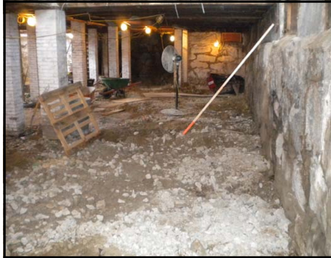
View of Basement floor slab demolition.
