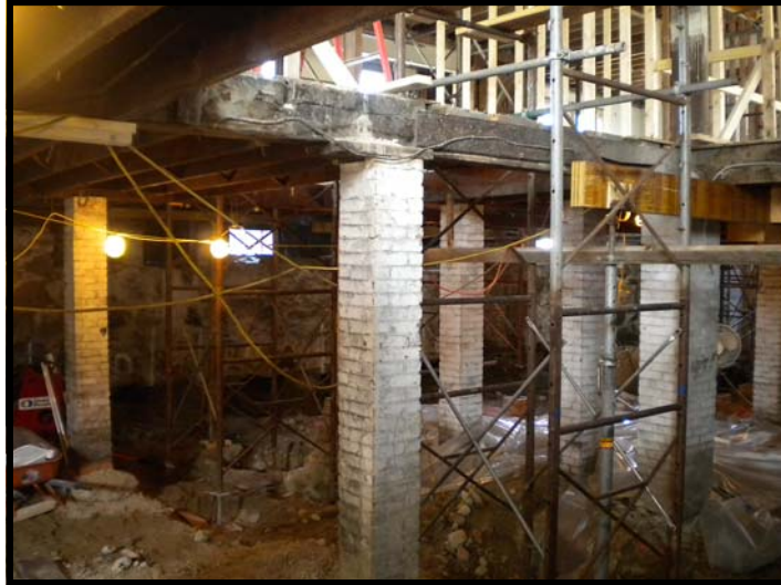
Basement view of former brick vault location during temporary shoring installation.
