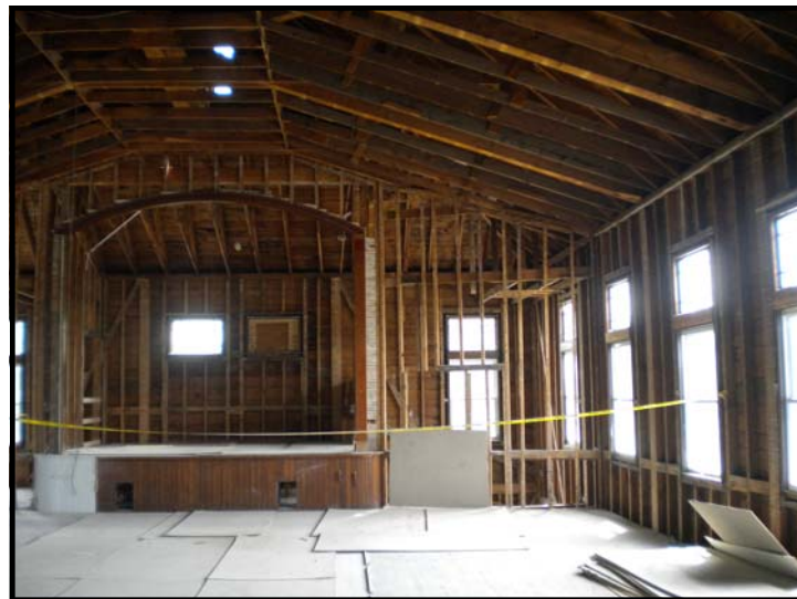
View of complete 2nd floor demo.
