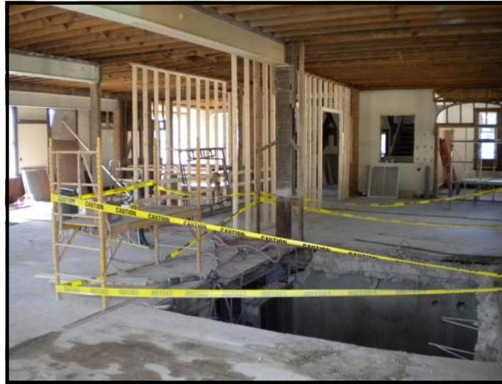
View of completed 1st floor vault demo.
