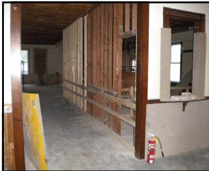
1st floor view post-demolition.
