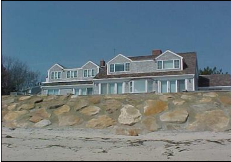
The surface of the rocks in this sloping revetment is relatively smooth and the spaces between the rocks have been filled with cement, further smoothing the structure. Smoother surfaces such as this reflect wave energy outward onto the beach and upward toward the house rather than dissipating the energy. The results are increased overtopping of the wall by waves, resulting in erosion and storm damage. (Photo: CZM)
