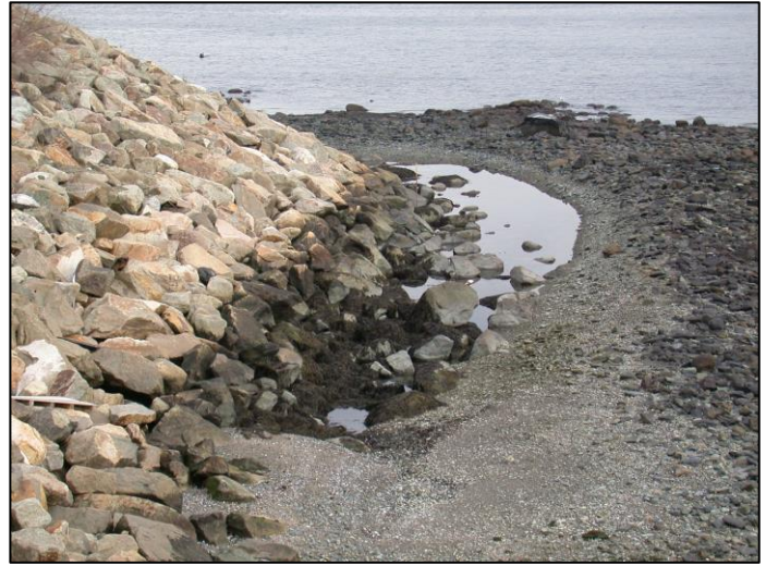
Erosion of the beach in front of this revetment created a depression at the base of the structure. (Photo: CZM)
