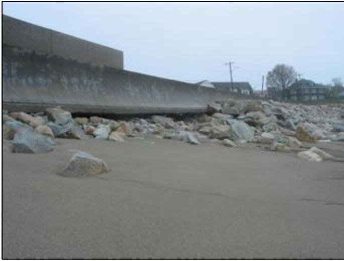
The beach in front of this concrete seawall eroded, undermining the structure. (Photo: CZM)
