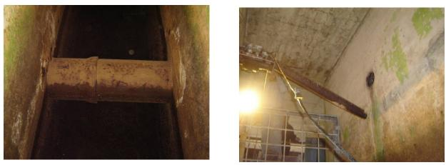
An abandoned, heavy rusted, 4" diameter steel conduit spans between the southerly and center walls, on the easterly side of the trash racks, approximately 12 feet above the invert slab and offset 3 feet west of the sewer line below. This conduit within the northern barrel of the sluiceway is broken and hanging from the center wall (shown on right above).
