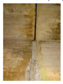
located in the wall. In addition, it appears that the construct joint has opened by approximately 3" at the bottom of the roof slab. As a result, what appears to be the waterproofing membrane, placed on the top of the roof slab, is clearly visible (shown on
