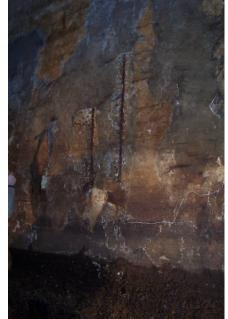
there is a heavy coating of barnacle and marine growth preventing a detailed visual inspection of the lower portion of the wall. In general, the south face of the center wall of the sluiceway is in fair to poor condition having experienced a higher state of deterioration than the south wall.
