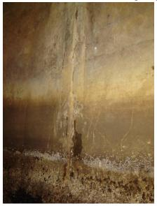
approximately 4'-6" above the invert slab and within the patch material either side of the vertical expansion joint. At this location, the patch material has lifted away from the wall. Similarly to the south wall, the vertical expansion joint has appeared to have opened up by approximately 3" at the bottom of the roof slab (shown on right below). However, unlike the south wall, the patch material filling the joint
