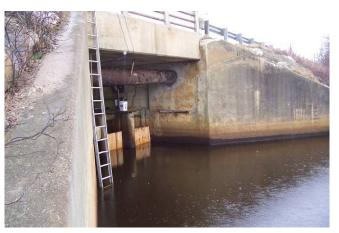
A 24" sewer line (shown on left below) spans between the northerly, center and southerly wall of the sluiceway, on the easterly side of the trash racks, and is located approximately 3 feet above the invert slab to the bottom of the sewer line.
