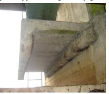
spalling along its bottom edges (shown on left below). However, the catwalk perpendicular extending between the inside faces of the wingwalls had extensive areas of spalling concrete exposed and steel reinforcement (shown on right below).
