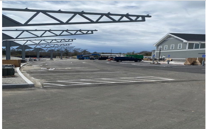
Solar Canopy install and Parking Lot striping in progress
