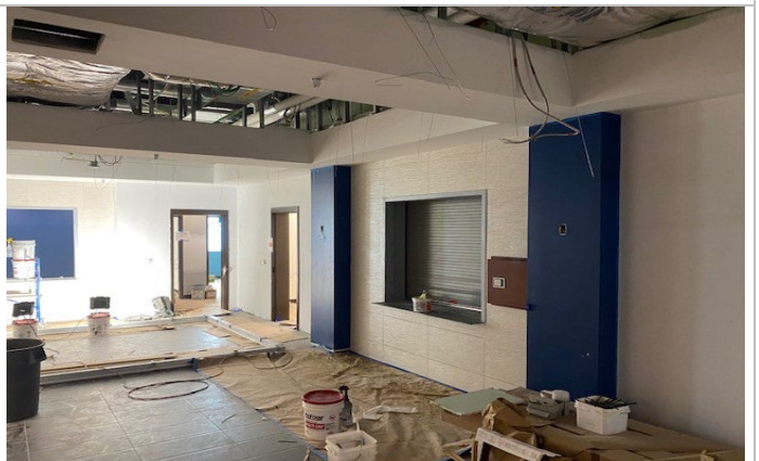
Tile install at Dispatch Wall
