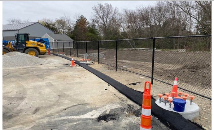
Asphalt Curbing and Fencing installed at Parking Lot
