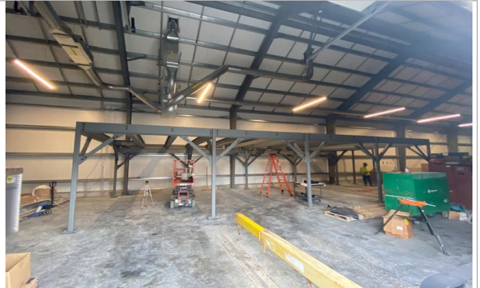
Mezzanine construction in progress
