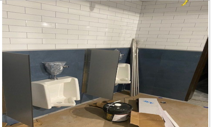
Bathroom fixture and partition install
