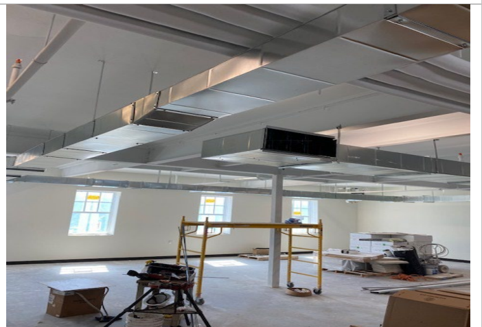
Ductwork at Storage area installed
