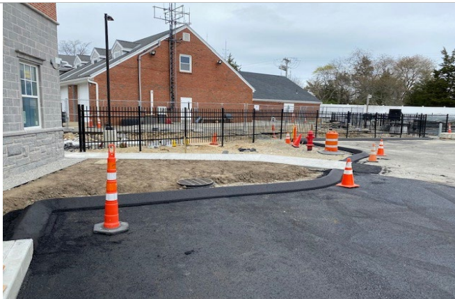
Asphalt curbing installed at Parking Lot
