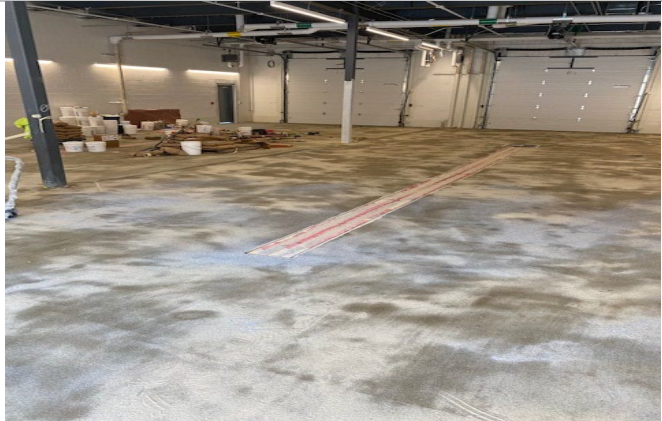
Sallyport floor prepped for epoxy
