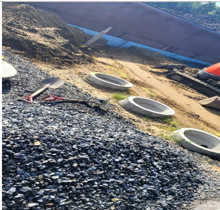
alt. view of tank tops being backfilled after being sealed and parged
