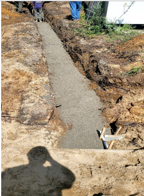
Tank at leaching field, covers sealed and backfilled with concrete
