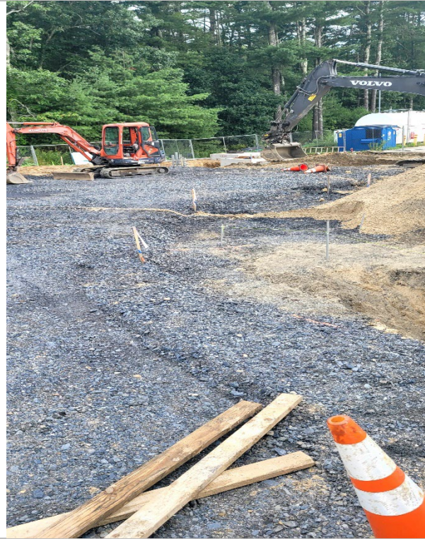
lt. view of leaching field and tank area being subgrade
