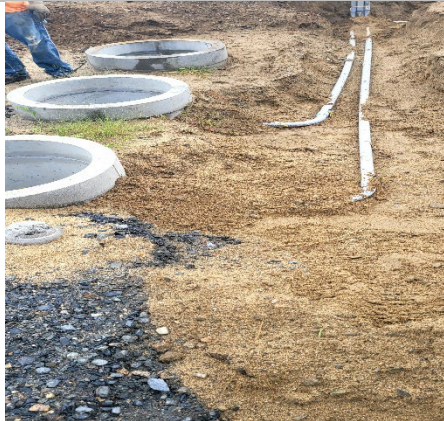
tank at leaching field, tops being parged and sealed with concrete
