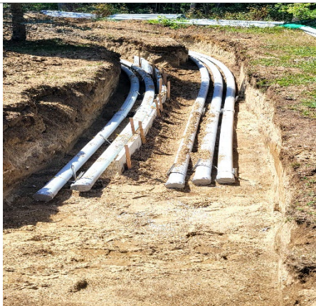
3 pipes are tele., 2 are elec, eventually lead to new pole.
