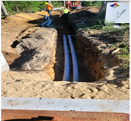
Electricians laying electrical conduit from transformer pad
