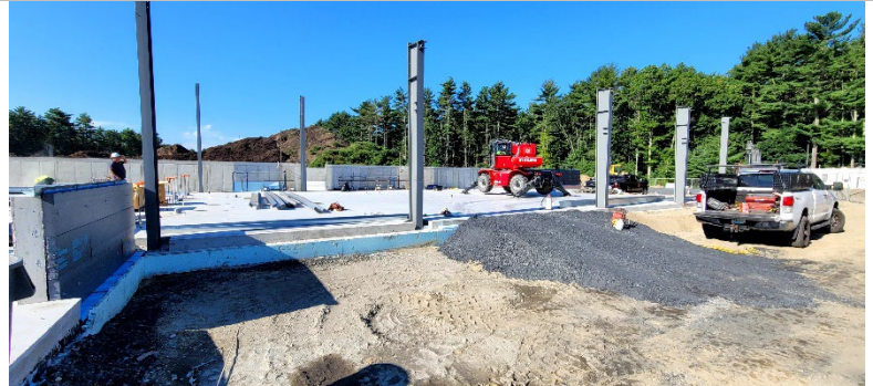
Start of steel columns being erected
