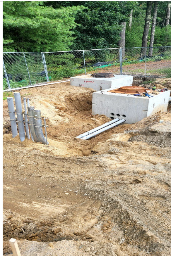
transformer pad, electrical conduit connected
