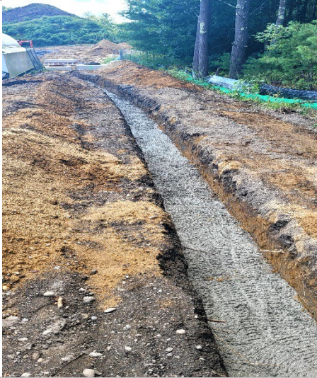
alt. view of tele data trench encased
