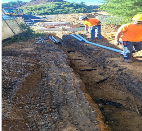
Electricians laying electrical conduit from transformer pad
