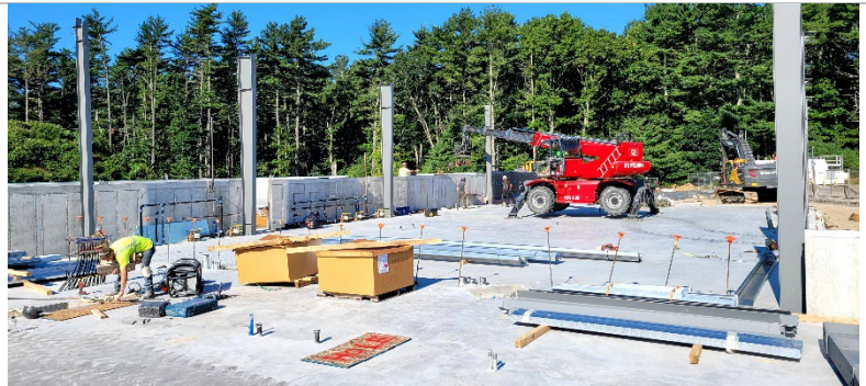
Start of steel columns being erected
