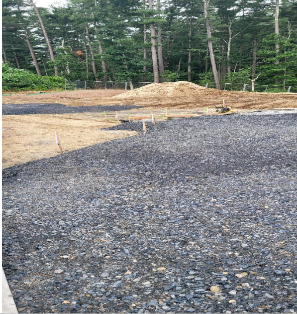
leaching field and tank area, being subgrade
