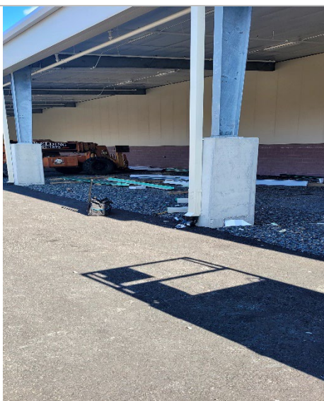
Downspouts installed at canopy area in rear of building
