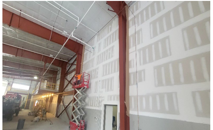
Demising wall in vehicle storage being taped and plastered
