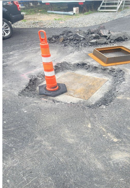
Remaining manhole covers being installed around the site
