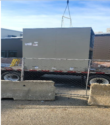
Another section of the generator being hoisted
