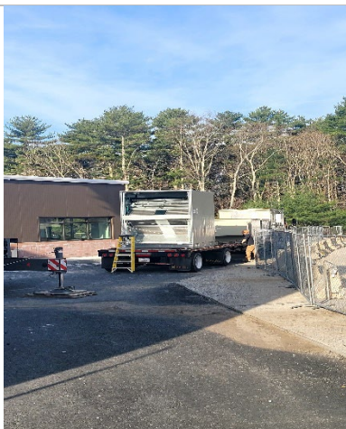
HRV-1 delivery to be installed on admin. roof
