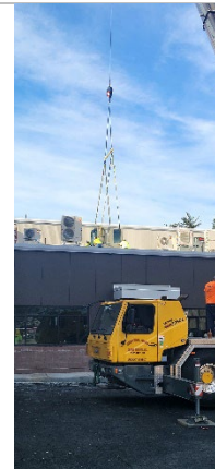
Crane hoisting HVAC generators onto admin. roof
