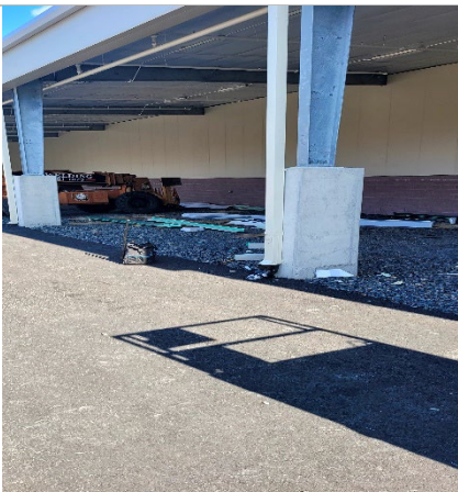
Downspouts installed at canopy area in rear of building
