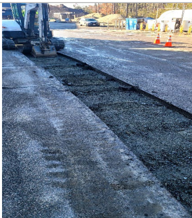
DPW backfilling gas line trench
