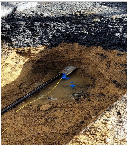
Gas line into sleeve
