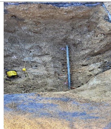
Gas line sleeve at T-line
