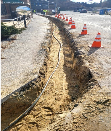
Gas line connected to sleeve
