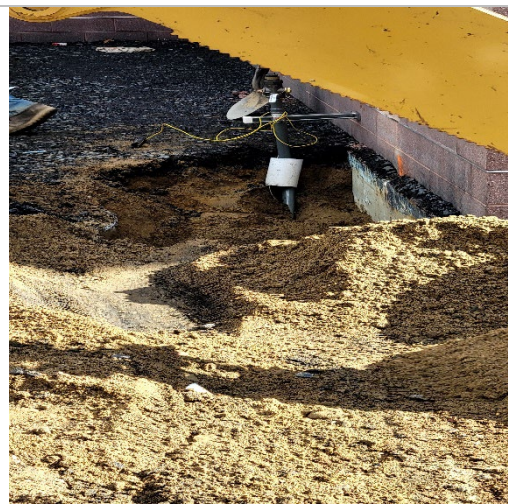
Gas line into new building at meter location
