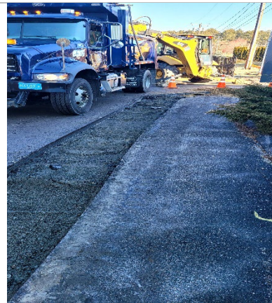
Trench for gas line back filled by DPW
