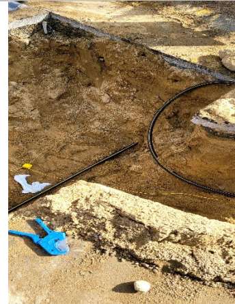
Gas line connected at T line
