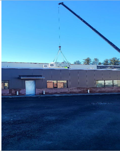
HVAC condensers being installed on admin. roof
