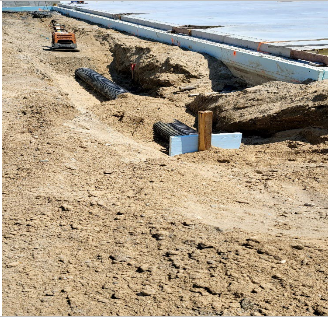
drainage pipe, capped at line 5A
