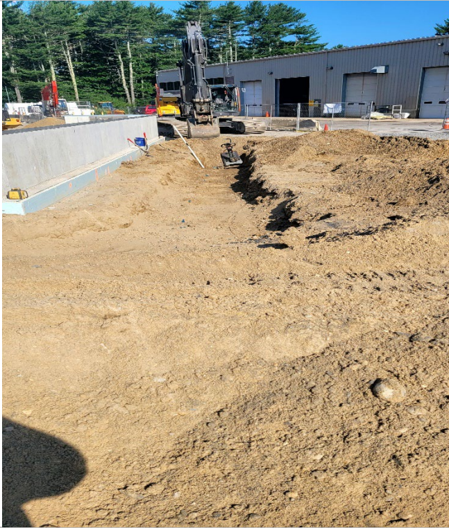
pipe install along exterior of building for downspouts
