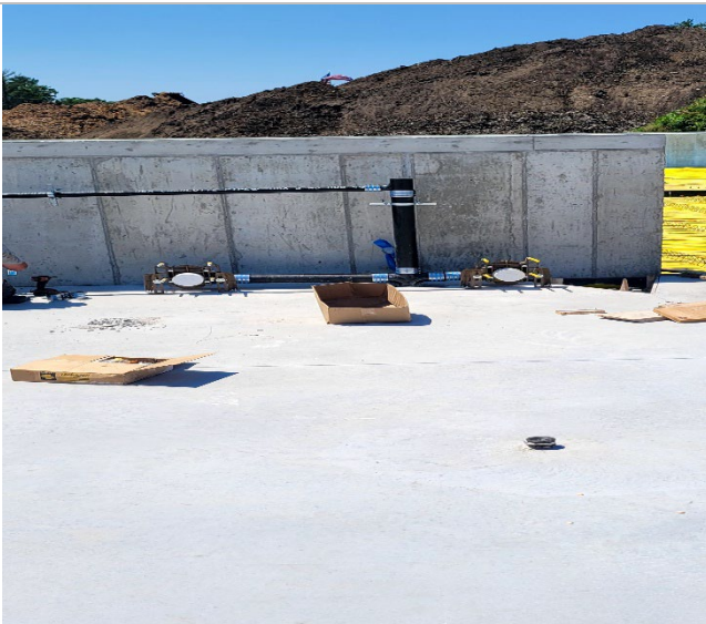
pipe install along exterior of building for downspouts
