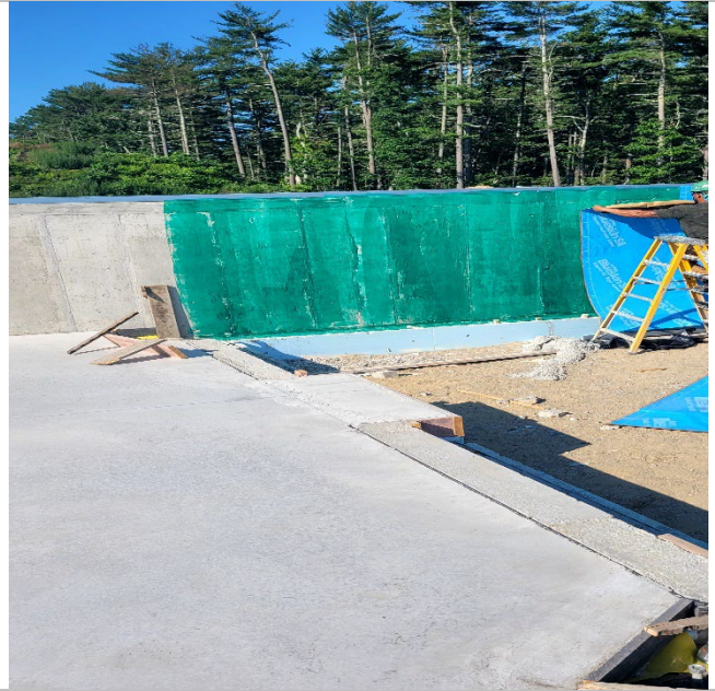
foundation knee walls being damproofed
