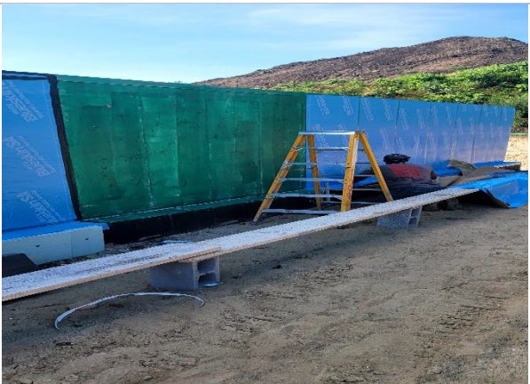
remaining wall along line 8A for waterproofing (AVB)
