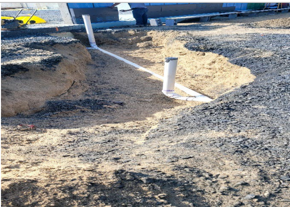
septic tank pipe for inspection
