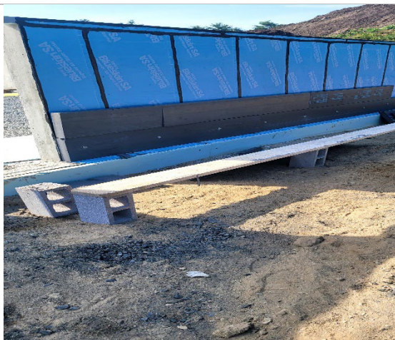
foam along wall 8A for masonry block
