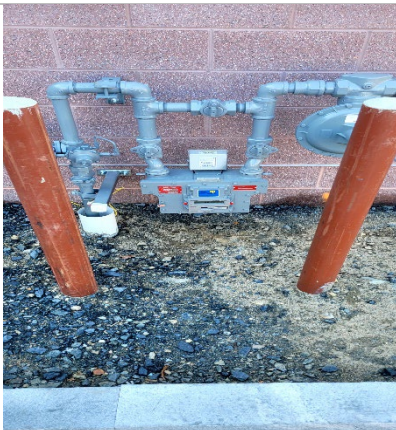
Gas meter installed outside of building.
