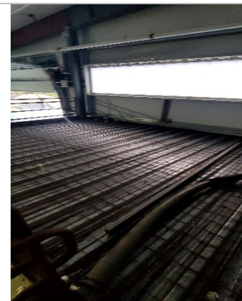
Alt. view of mezzanine in vehicle storage prior to concrete pour
