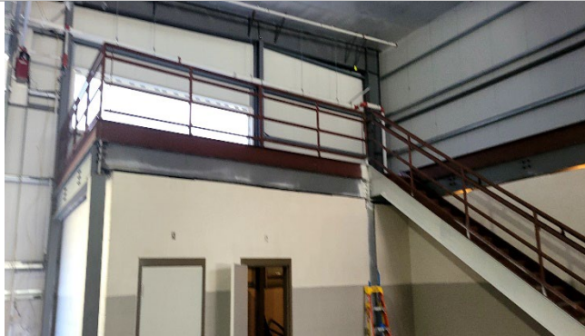
Stairs and railings leading to mezzanine in vehicle storage
