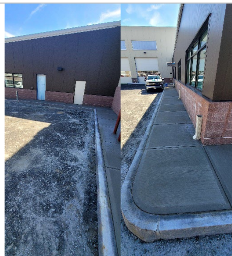
Alt. views of the sidewalk after concrete pour.
