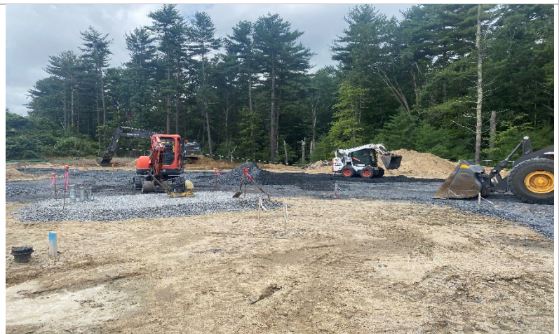
Site crew, compacting area for future spot of generator
