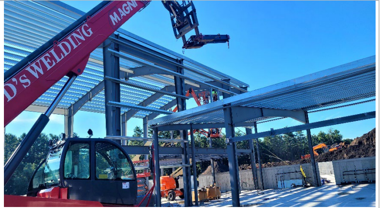
Side trim and clips being installed
