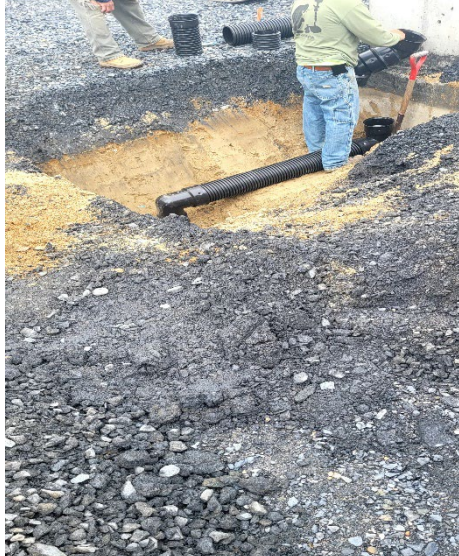
Roof drainage pipe being installed
