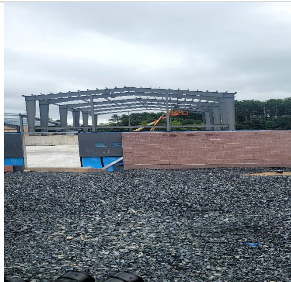
Alt. view of roof purlins being erected
