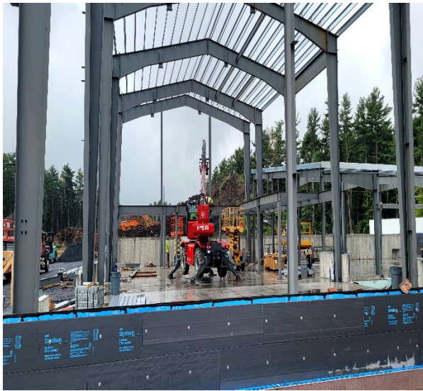
Mezzanine level being erected
