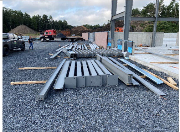
Steel beams laydown area
