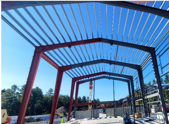
Vehicle maintenance painted and coated, with roof purlins installed
