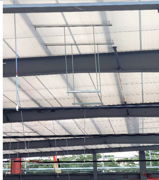
Hangers installed in vehicle maintenance for duct work
