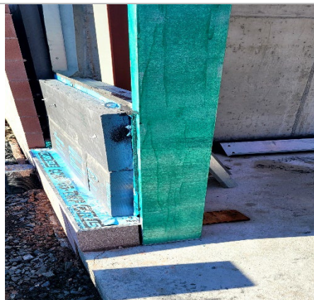
Another doorframe with waterproofing sealant
