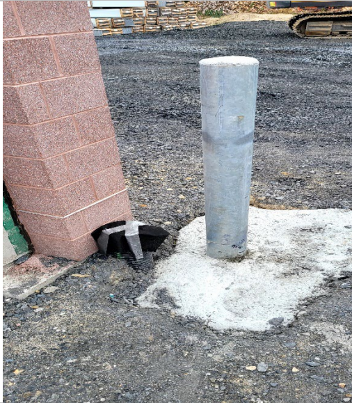
Steel bollards installed and filled with concrete
