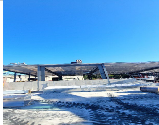
Rear view of admin. building w/ roof fabric and panels beginning to be installed
