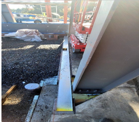
Metal track installed to begin framing walls
