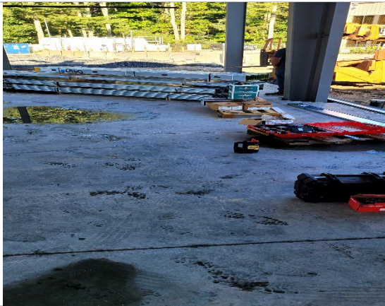
Metal track and studs ready to be framed
