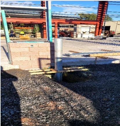
Bollards being installed at all doorways
