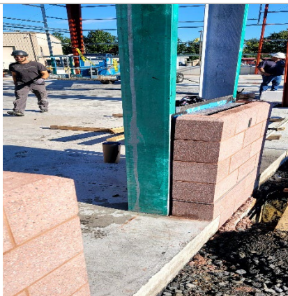
Doorframes being coated with waterproofing sealant
