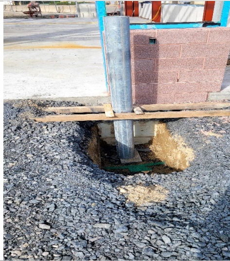
Bollards being installed and braced before concrete pour
