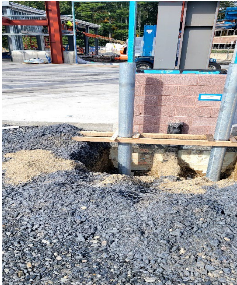
Bollards at garage bay being prepped for concrete pour
