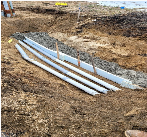
Conduit from existing pole to new pole before being backfilled
