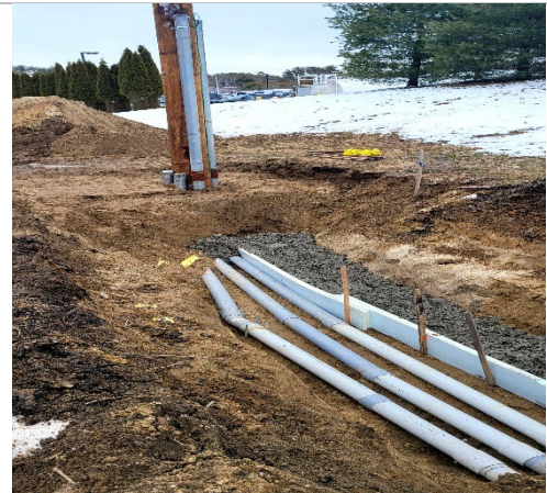
Another view of conduit to new utility pole
