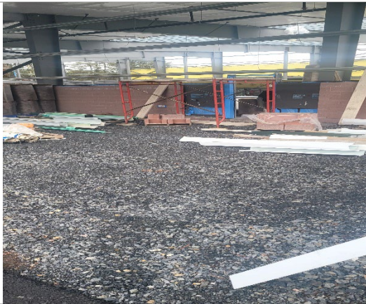
Scaffold set up for exterior masonry work
