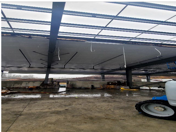
Roof banding and clips, along with insulation in vehicle storage
