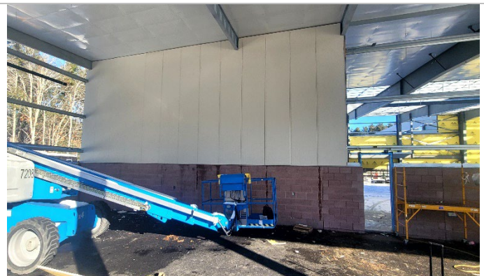
Wall panels being installed in canopy area
