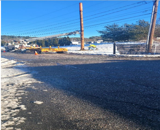
Pole being held in place by Verizon
