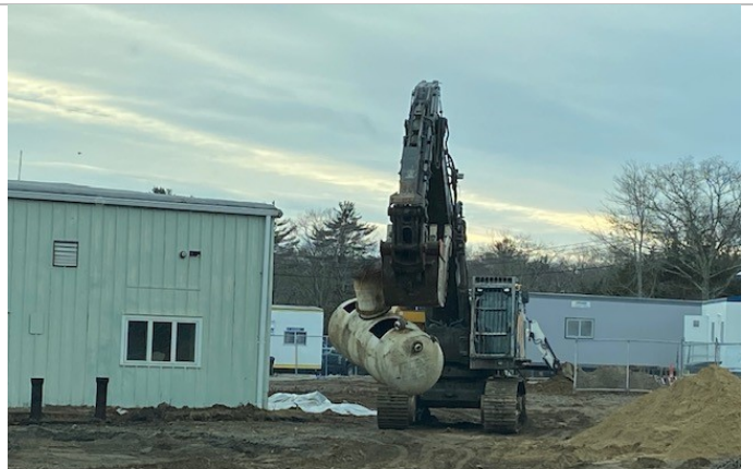
Removal of Holding Tank
