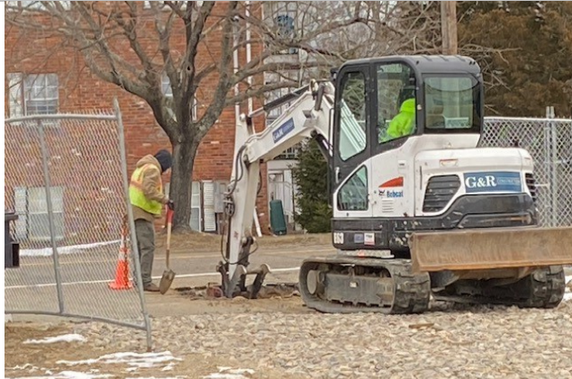
Excavation for Cutting and Capping of Sewer Main
