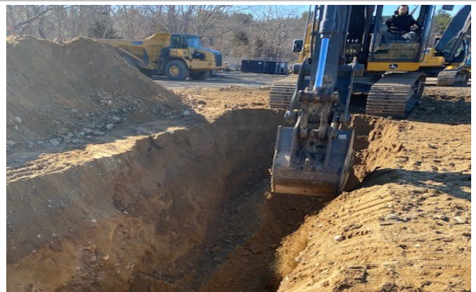
Test Pit excavated at Hydraulic Lift Area
