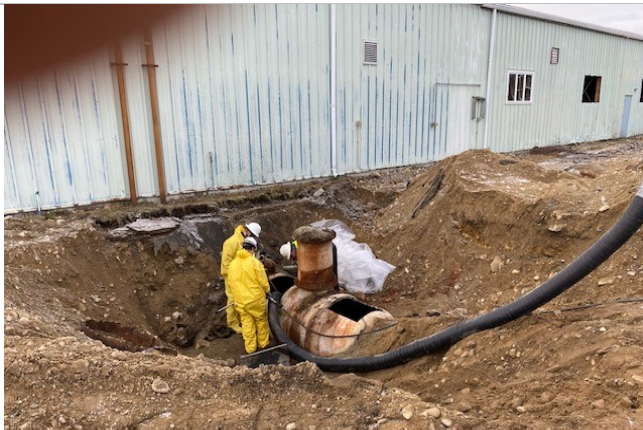
Vacuuming of 1,000 gallon Holding Tank prior to removal and demolition
