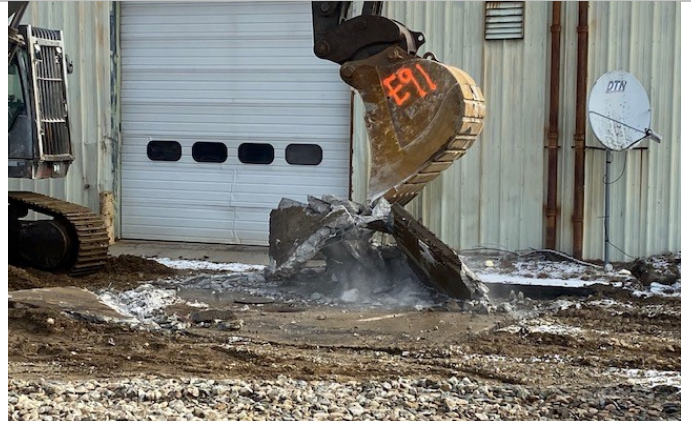
Demolition of Concrete Pad for access to pump, remove, and demolish 1,000 gallon Holding Tank
