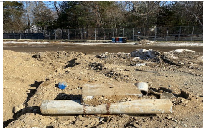
Transite Pipe uncovered during course of Slab Demolition
