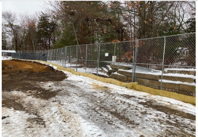
Erosion Control Installed along Site Fencing
