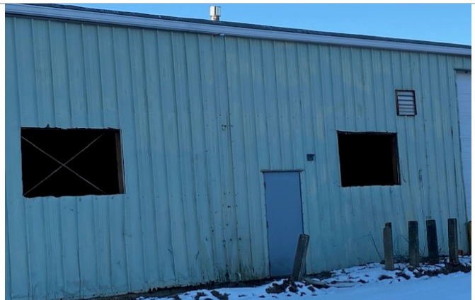
Windows Removed from DPW for PCB Abatement
