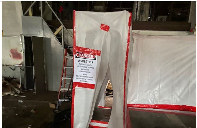
Ante Room Constructed for Asbestos Abatement
