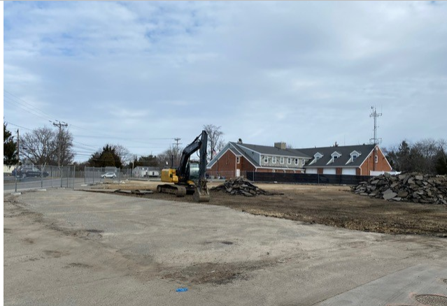
Existing Asphalt Parking Demolished and Stockpiled for Removal from Site
