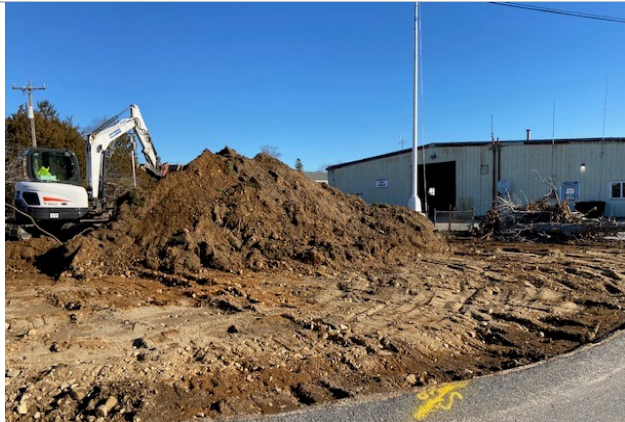
Clearing and Grubbing at Southwest Corner for Temporary Parking
