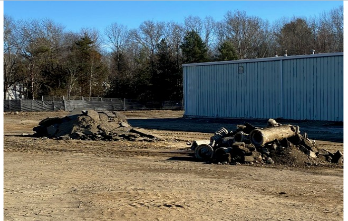
Existing Storm Drainage Removed and Demolished
