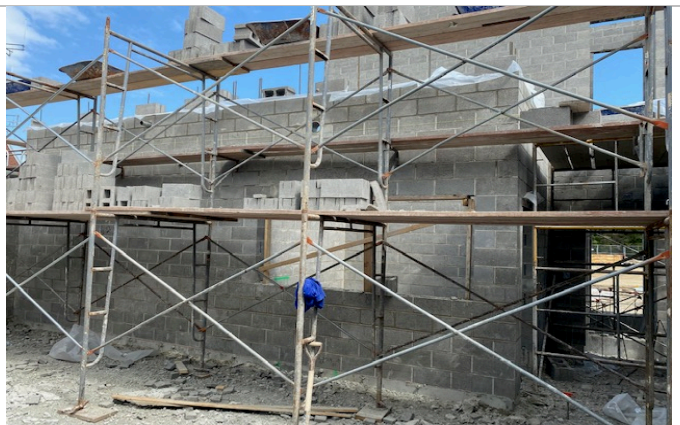
Inside view of CMU work in Dispatch Area
