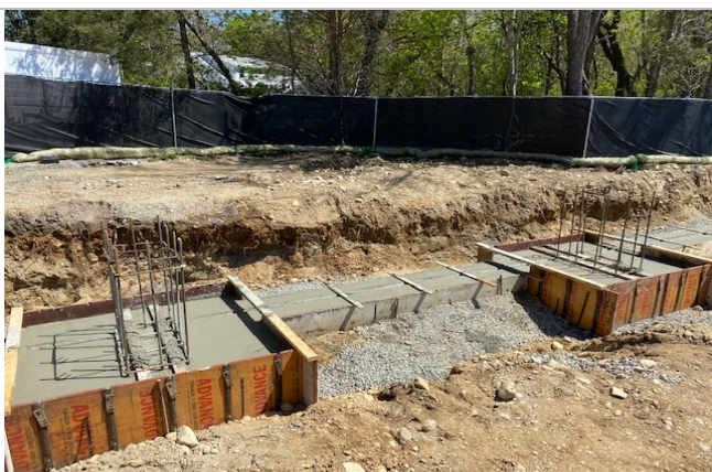
Concrete placed for footings at Auxiliary Building
