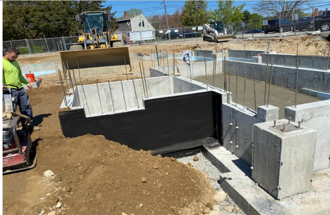
Installation of Waterproofing and Backfill and Compaction at Elevator Pit
