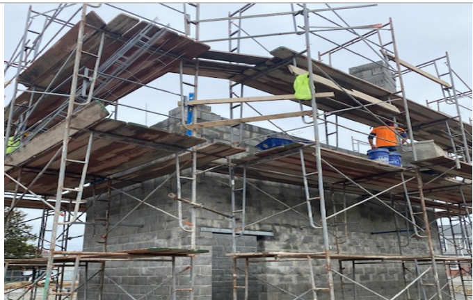
Lintel installed at Doorway at Stairway 12
