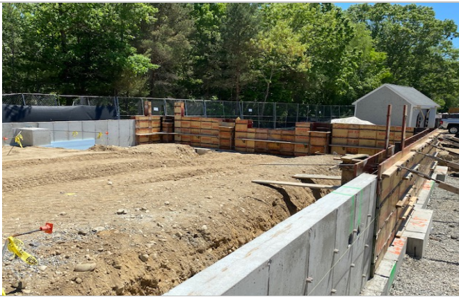
Forming of Foundation Walls at Auxiliary Building
