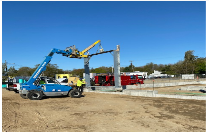
Installation of Sallyport Door Frame
