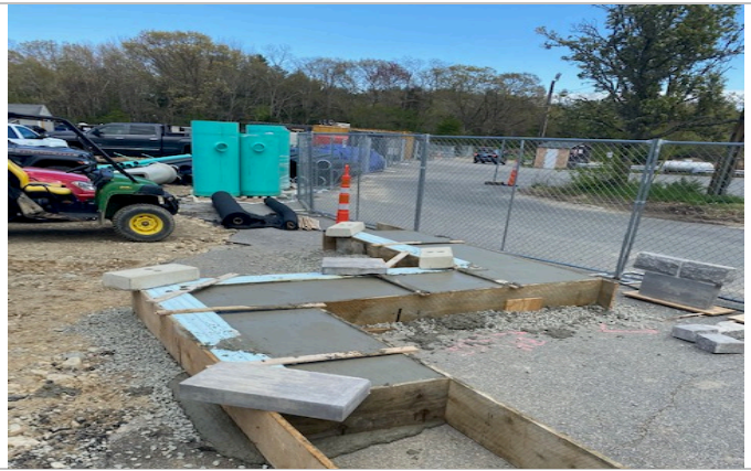
Forming of Foundation for Masonry Mockup
