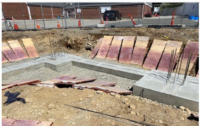
Footings at Auxiliary Building stripped
