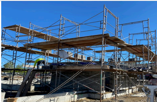
Scaffold Erection and Ongoing CMU at Stairway 12
