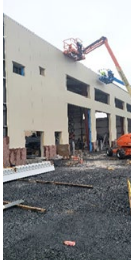
Side panels being installed on vehicle maintenance building
