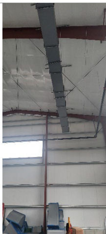
HVAC in vehicle maintenance building
