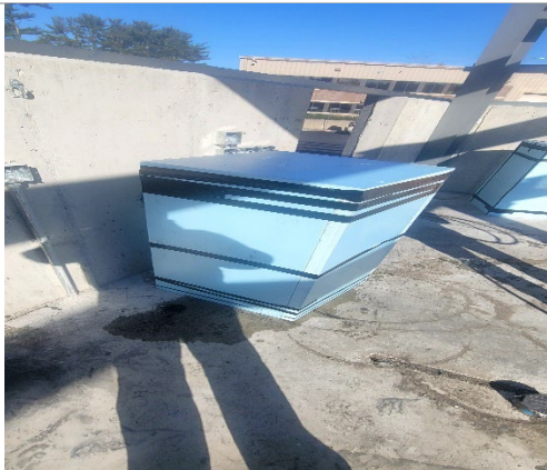
Electrical room in vehicle storage building, stub ups being protected
