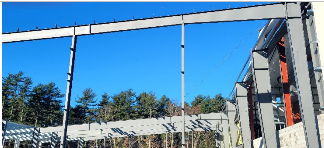
Steel columns and mezzanine being erected in vehicle storage
