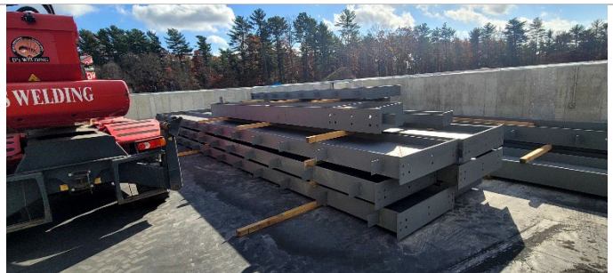
Steel columns in vehicle storage area
