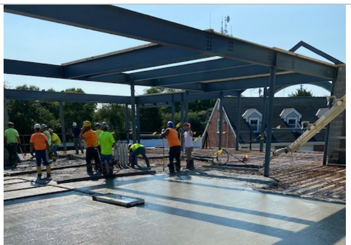
Concrete Placement at 2 nd Floor Slab On Deck
