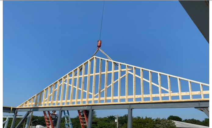
Roof Truss set in place at Column Lines 2-4
