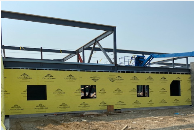
Densglass installed at Column Lines 8-10 at Parsonage Street side
