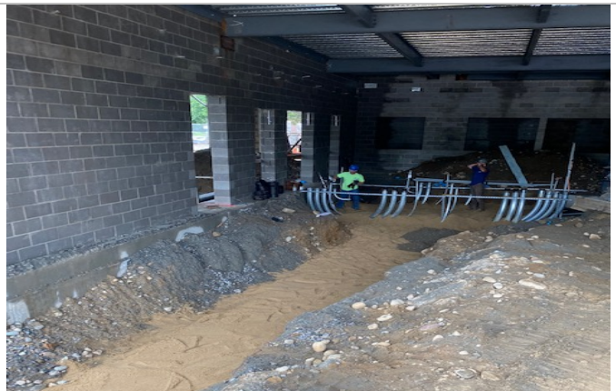
Trenching for Underslab MEP's between Column Lines 2-3
