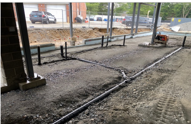
Underslab plumbing installed at Lobby for Men's and Women's Bathrooms
