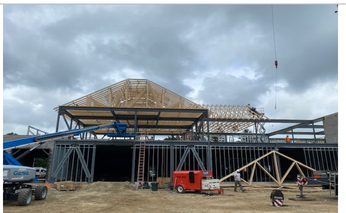
Ground view of Roof Truss progress
