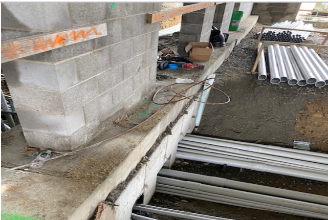
Underslab Electrical Installed at Column Line 2 into Police Station
