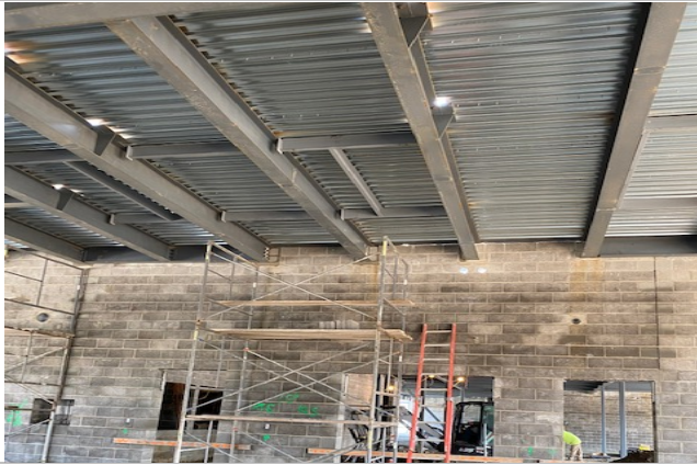
Infilling of Beam Pockets at Sallyport
