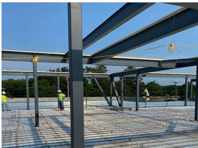
Installation of Chairs and Wire Mesh in preparation of Slab on Deck Pour
