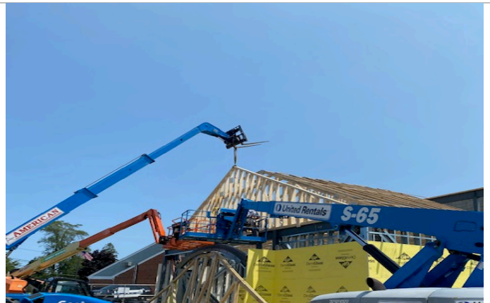
Roof Trusses being installed at E.O.C. (ground view)
