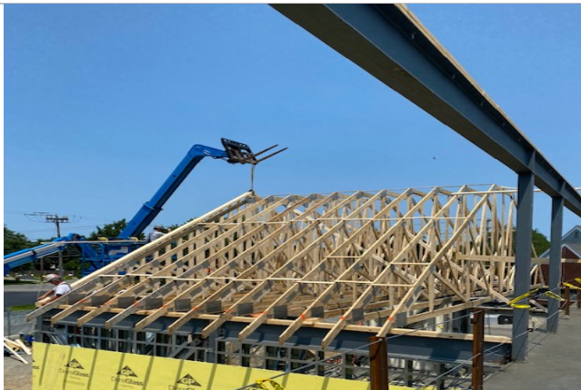
Roof Trusses being installed at E.O.C. (2 nd Floor view)
