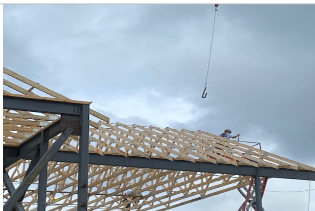
Roof Truss installation from Column Lines 4-9 underway
