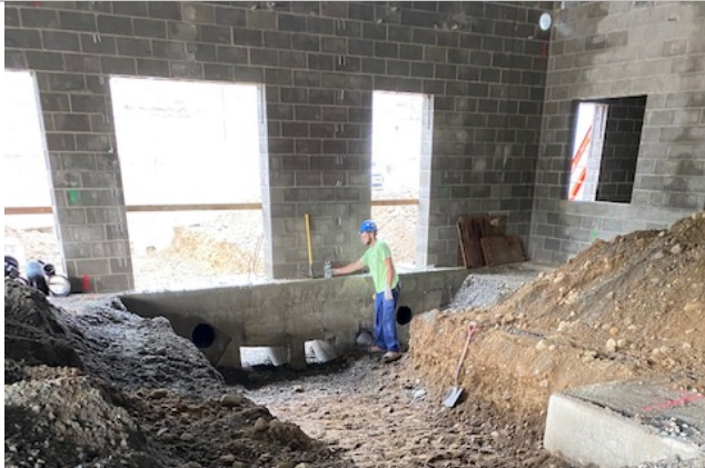
Trenching for Installation of Underslab Electrical at Sallyport
