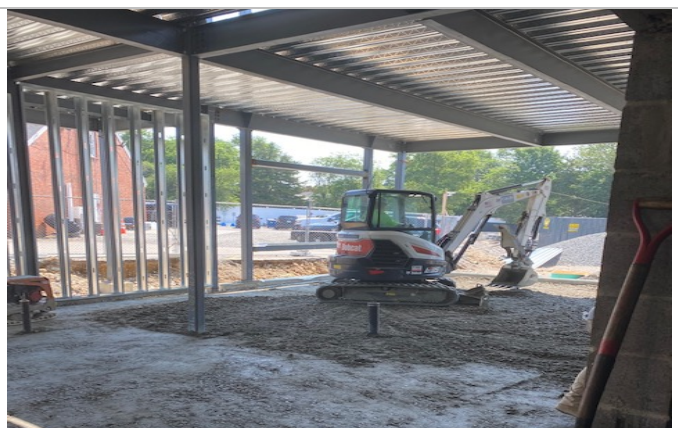
Backfilling and compaction at Lobby Area
