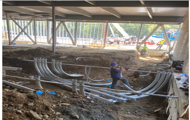
Installation of 4" conduit for Primary Electrical
