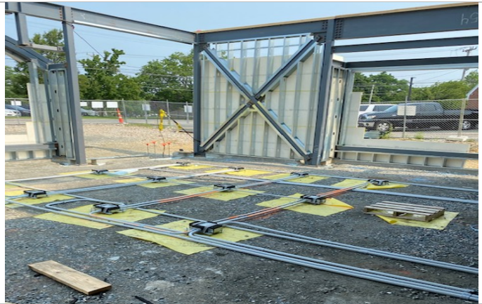
Installation of Floor Boxes and Conduit in E.O.C.
