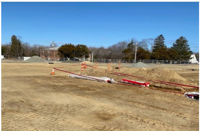
Removal and Abatement of Transite Pipe
