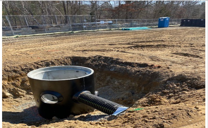
DMH – 3 with HDPE pipe install and backfill complete
