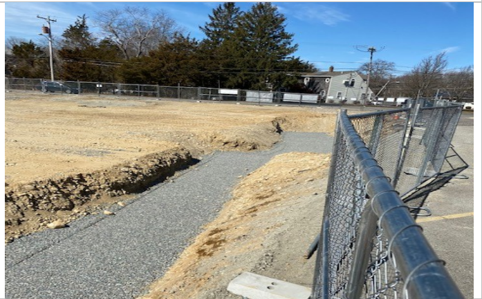
Crushed stone installed and proof-rolled at Northeast corner of site
