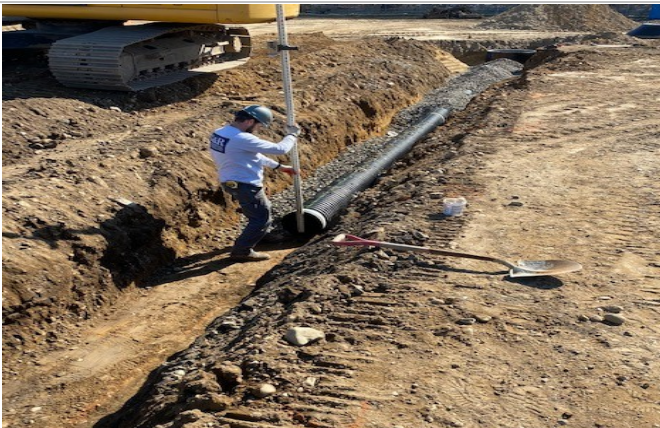
Grading of pipe installation and continuation of drainage line
