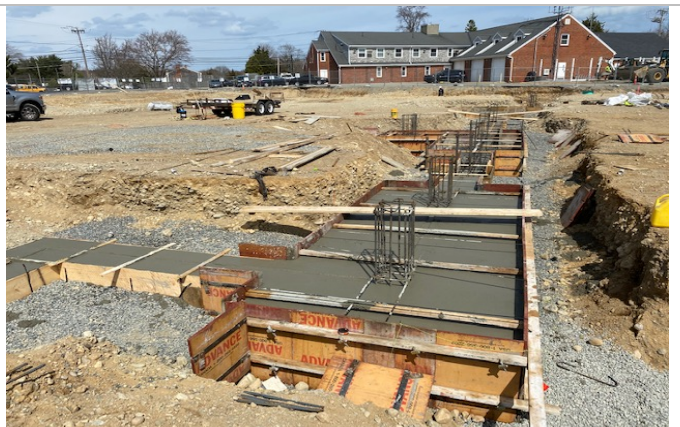
First Concrete Pour for Exterior Foundation Completed
