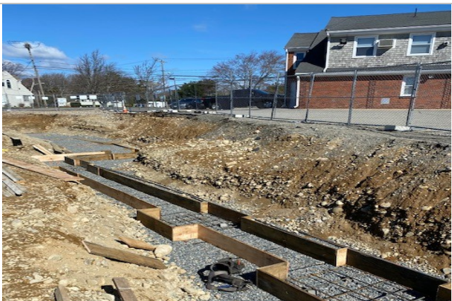
Installation of rebar at Eastern side of Building
