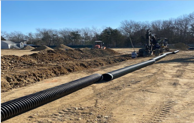
Layout of HDPE pipe prior to installation from DMH – 3 to DMH - 2
