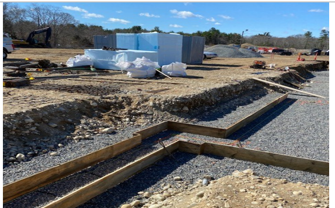
Forming of Foundation and Wall Footing along rear of Building
