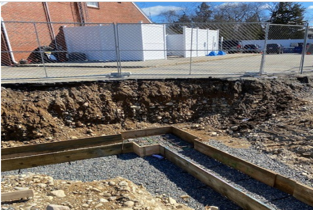
Formed Pier and Foundation at Southeast corner of Building
