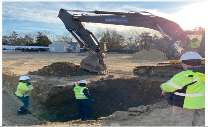
Testing for Contaminated Soils at Drainage Pit
