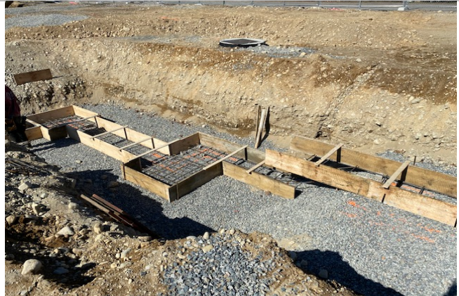
Formwork and Rebar Installed at Exterior Stepped Footing
