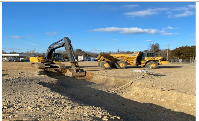
Excavation for Exterior Footings and Foundations at rear of building footprint
