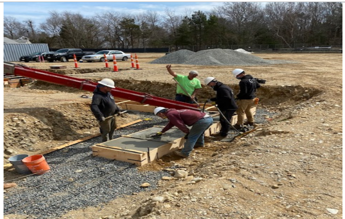
Placement of Concrete at Exterior Foundation
