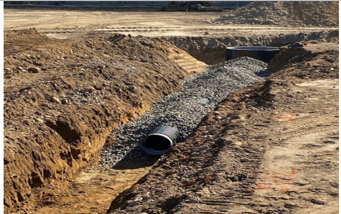
HDPE Pipe installation and installation of crushed stone
