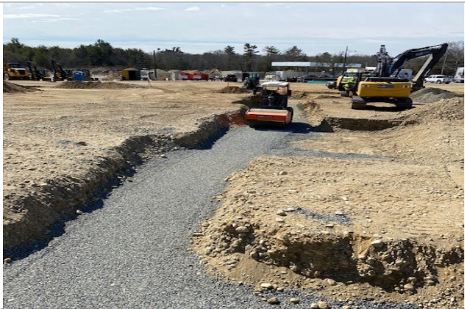
Installation and Proof-rolling of crushed stone at rear exterior foundation excavation
