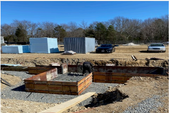
Forming of Footing at Rear of Building
