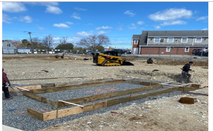
Forming of Wall Footing at Rear of Building
