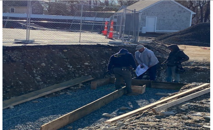
Formwork for Footings and Foundations Begin
