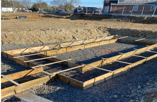
Rebar and Bracing installed at Wall Footing
