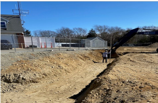
Excavation for Exterior Footings and Foundations at Northeast Corner of site
