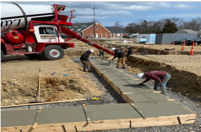
Concrete being tooled and finished
