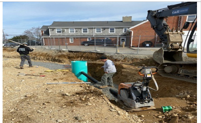
Installation of PVC Catch Basin – 5 at Southeast corner of building footprint
