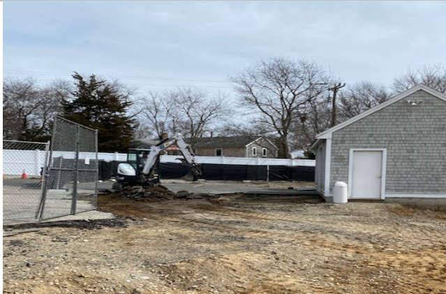
Demolition of asphalt in preparation of shed relocation
