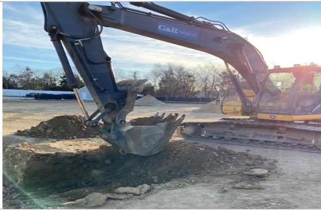
Excavation of Contaminated Soils at Drainage Pit
