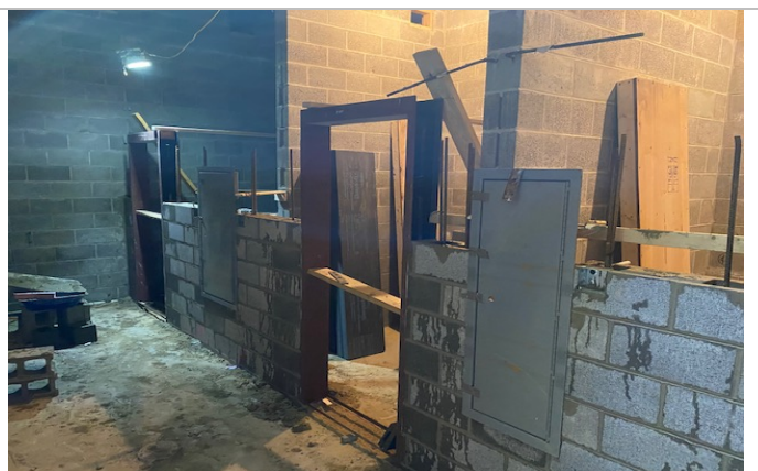
CMU construction and frame install at Men's Cells
