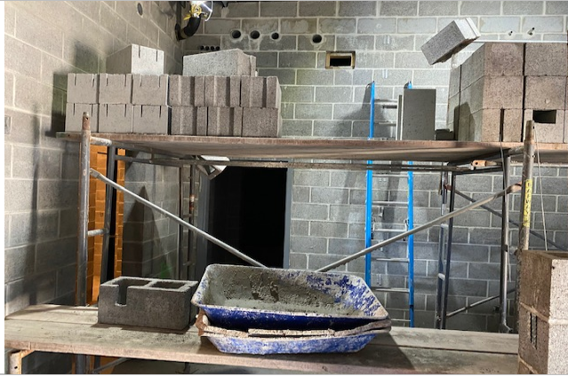
CMU Construction at exterior of Female Cells
