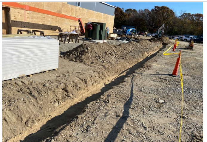
Trenching for Sewer Line for Auxiliary Building
