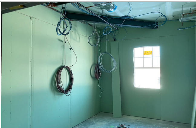
Drywall installed at Lieutenant's Office
