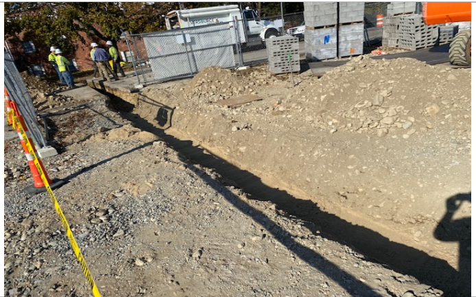
Trenching for Gas and Sewer from Parsonage Street
