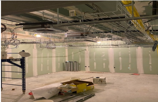
Wire trays installed at IT Server Room
