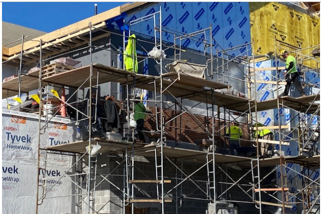
Exterior Brick install at rear of building
