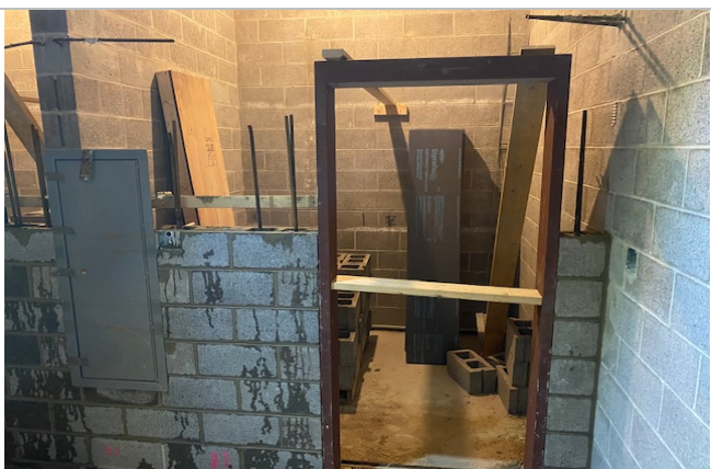
Detention Cell Frames installed
