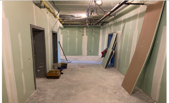
2 nd Floor Hallways Drywall and Taping completed
