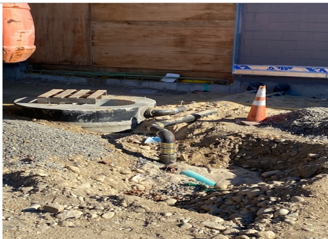
Piping installed at Oil/Water Separator at Sallyport
