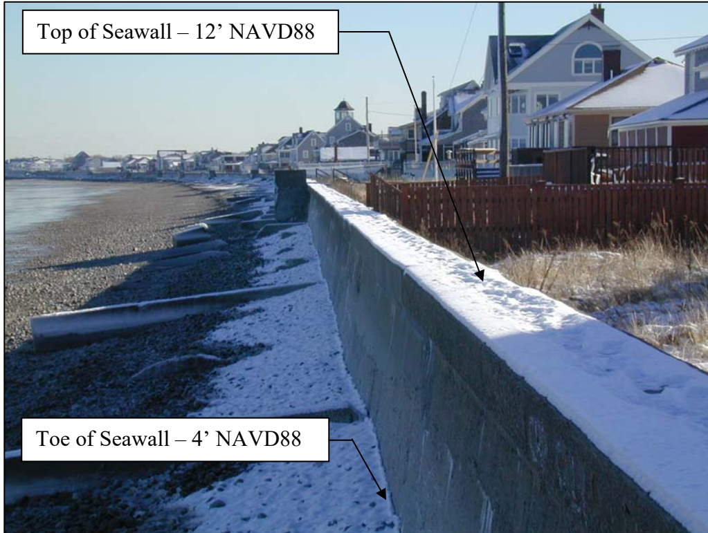
Figure 8. Representative seawall cross sectional picture
