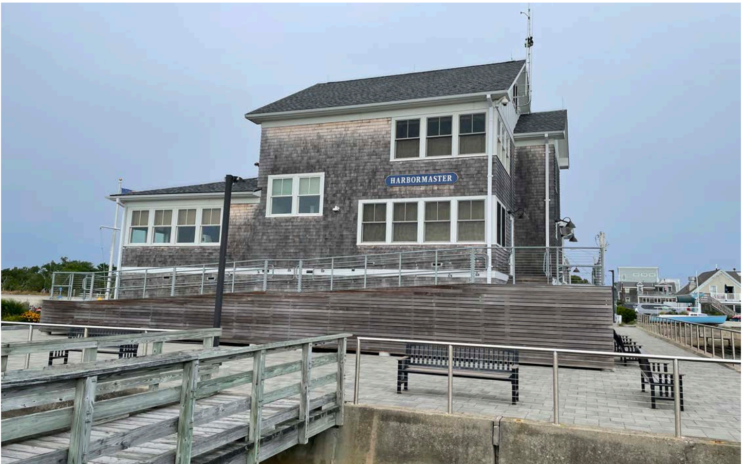
The Harbormaster Facility at the Town Pier. (Source: MAPC, 2022)
