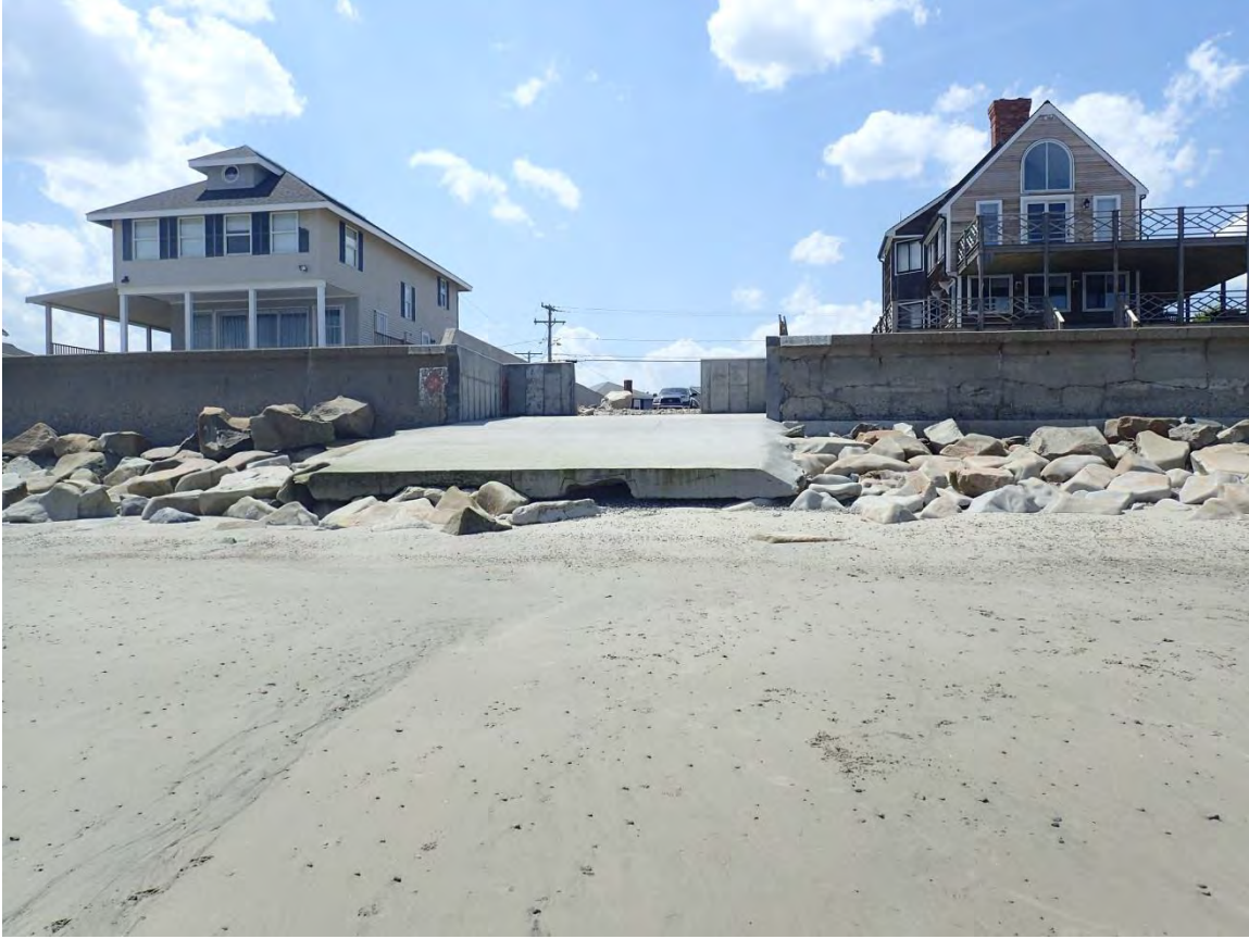
Figure 2-33. Vertical erosion and lowering of the beach elevation has caused exposure of the access ramp at the corner of Bay Ave and Bay St.
