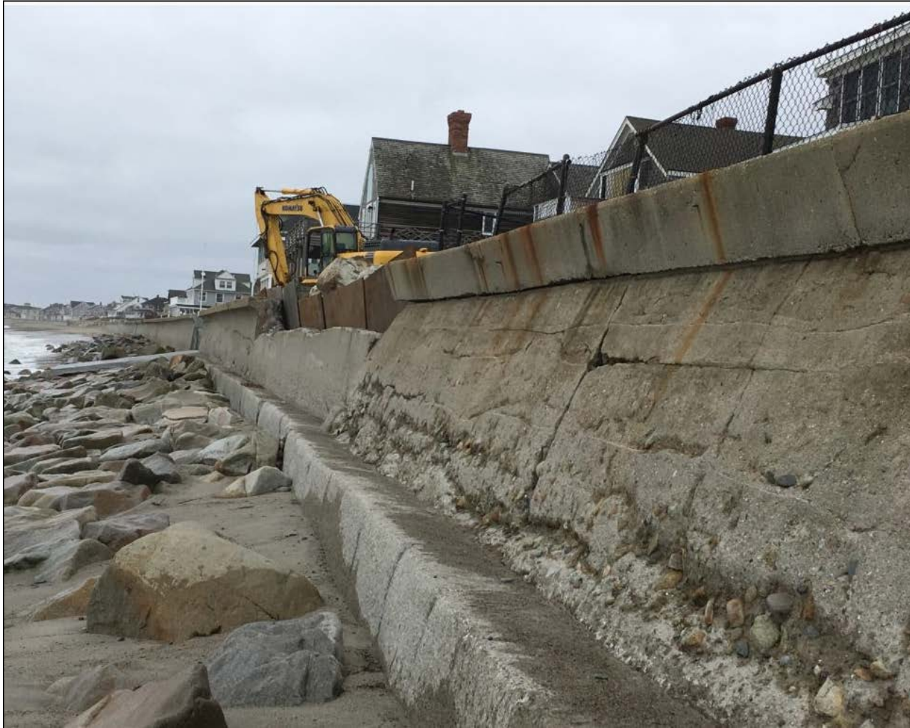
Seawall Failure and Property Damage
