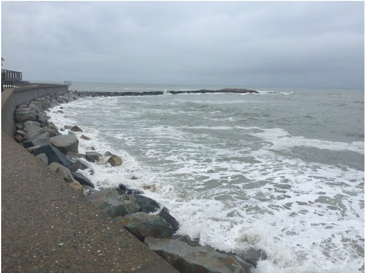
Figure 3-4. There is no dry high tide beach along much of Marshfield's coastline, including this location south of the main Brant Rock groin.
