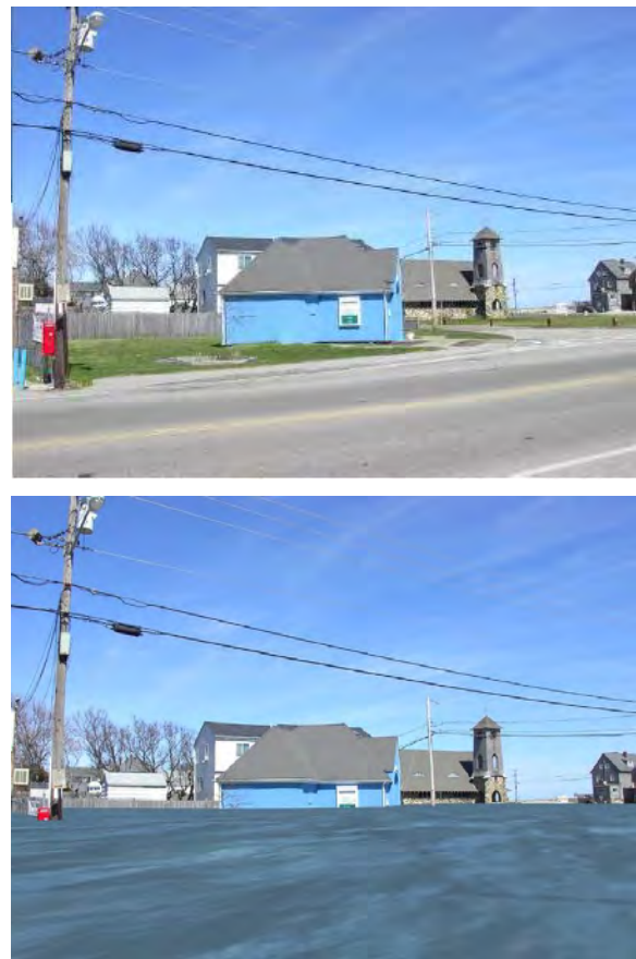
Figure 3-11. Beach comfort station at Brant Rock during present day (top) and by 2088 based on Kleinfelder’s sea-level rise projections (bottom).
