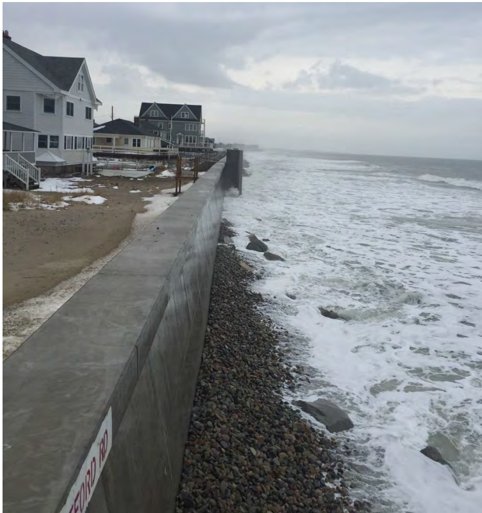
Figure 2-3. Fieldston Beach seawall (looking north from the end of Hartford Road).
