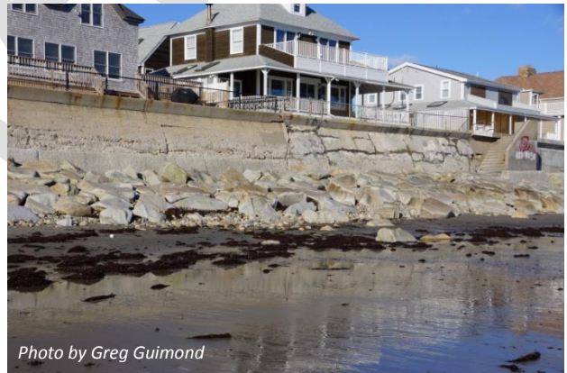
Sea wall along Bay Avenue
