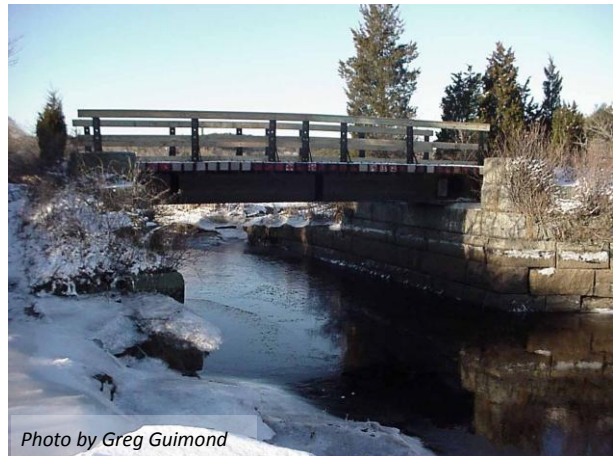
South River pedestrian bridge
