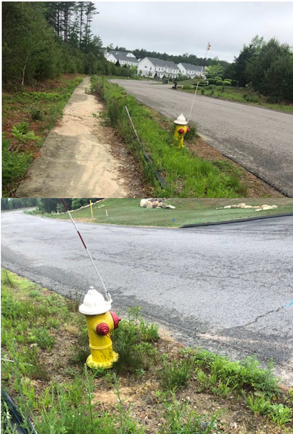
Commerce Way Fire Hydrants
