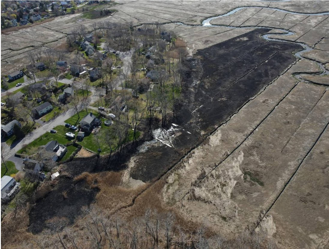
Figure 3-20. The aftermath of illegal burning which resulted in a marsh fire during the spring of 2022 on Anderson Drive in Marshfield.
