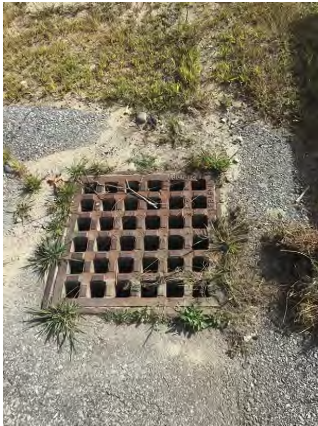
Oil/grease separator
