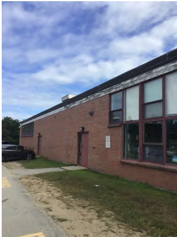
No gutters. Needs new roof
