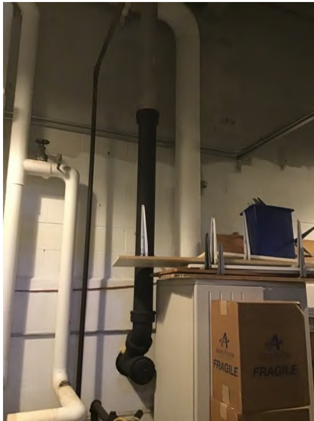
Tie in to roof drain
