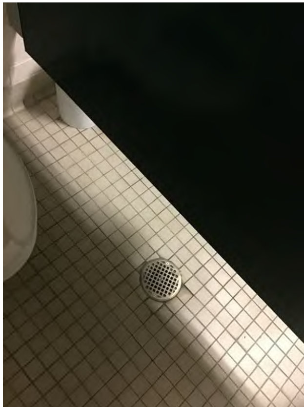
Bathroom floor drain
