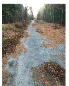
Trail section with deteriorating asphalt.
