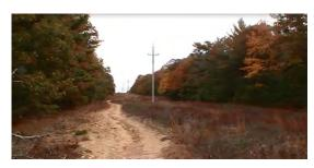
Graded Trail at Utility Easement. Recommend improving surface and/or rerouting trail to achieve more gradual slope.
